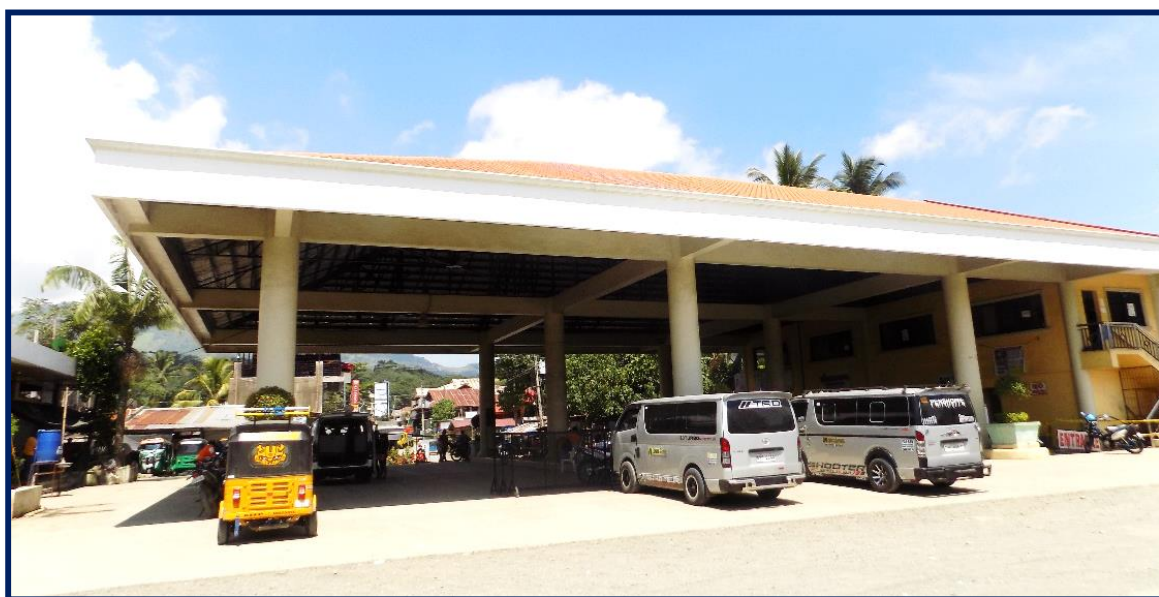
San Fernando Municipal Public Terminal
