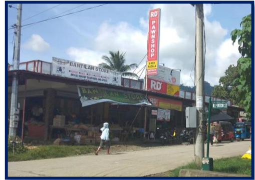
Hallasgo Commercial Building @ Purok 5, Halapitan (Hardware, Pawnshop, Optical Clinic, Ukay-ukay, Sari-sari store, Rice retail)
