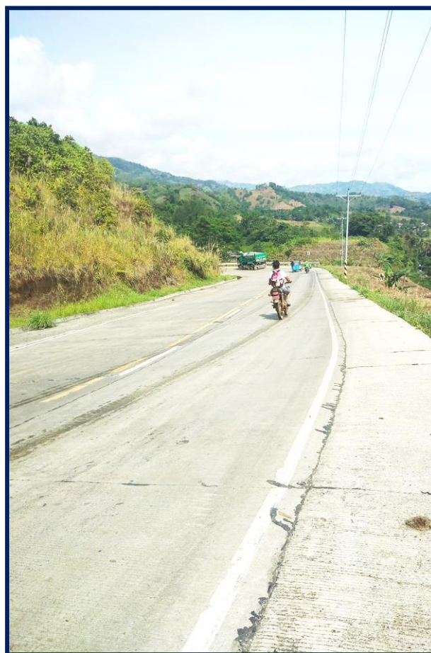
National Highway along Sitio Sulog of Barangay Halapitan
