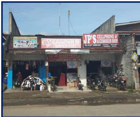
Onting Commercial Building @ Purok 6, Halapitan (Ukay-Ukay, Bakeshoppe, Cellphone Accessories)
