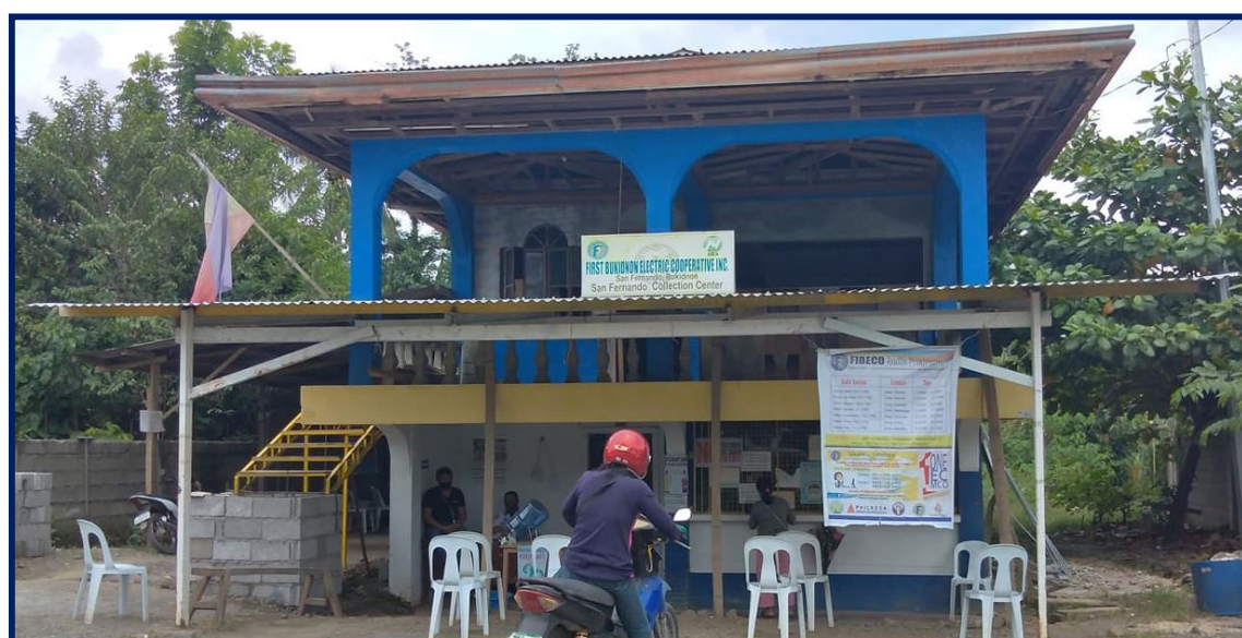
FIBECO San Fernando Collection Center @ Purok 1 of Barangay Halapitan
