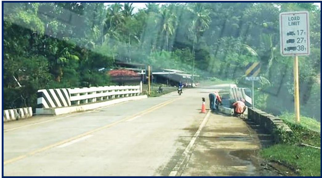
Mabuhay Bridge along National Highway at Barangay Mabuhay, San Fernando, Bukidnon
