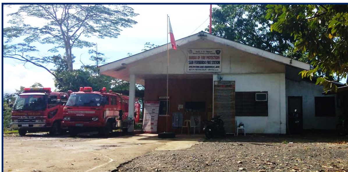
San Fernando Municipal Fire Station
