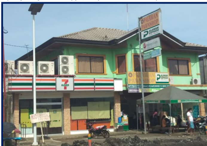
Navarro Commercial Building @ Purok 3, Halapitan (Convenience Store, Pawnshop, Rice Retail)
