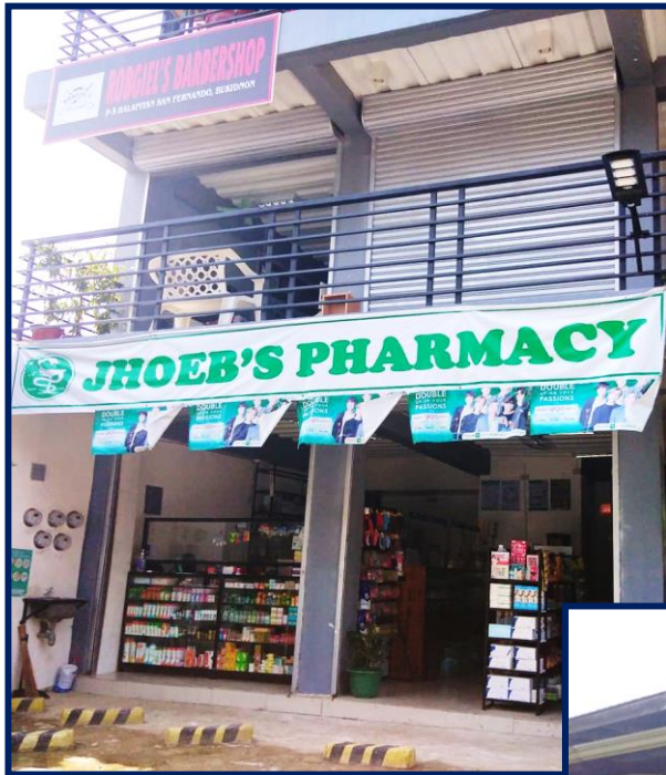
Paquiao Commercial Building @ Purok 5, Halapitan (Pharmacy, Barbershop, Restobar)
