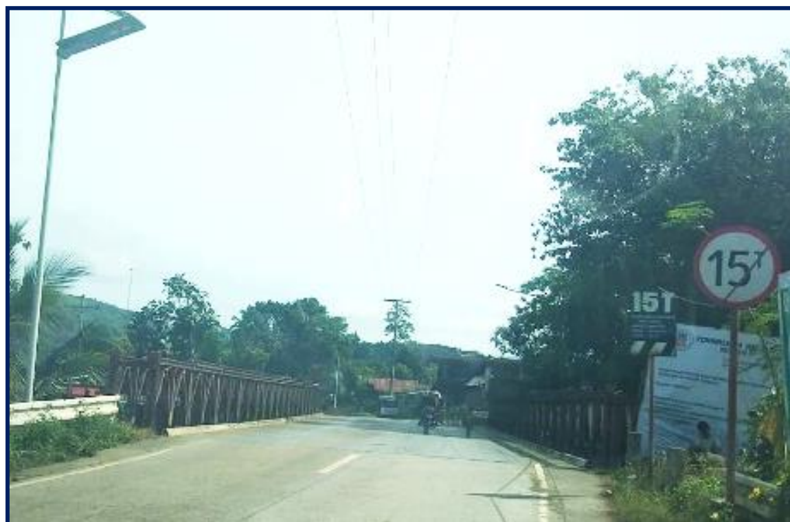
Mawie Bridge along National Highway at Purok 1, Poblacion, Halapitan, San Fernando, Bukidnon
