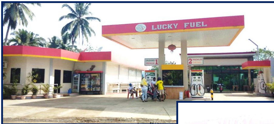
Lucky Fuel Gasoline Station @ Purok 9, Halapitan
